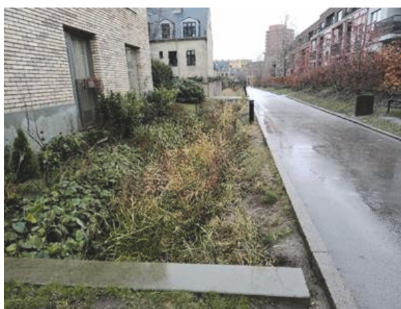
Fig. 3. An example of a rain garden/infiltration ditch from Copenhagen. A surface flow of stormwater can be collected in a trough with vegetation that withstands temporary flooding
