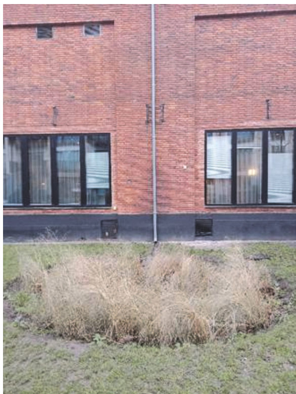
Fig. 2. An example of a rain garden/infiltration ditch from Copenhagen. An excess of stormwater from the roof is collected in a trough with grass vegetation
