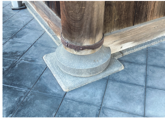
Fig. 4. Column base placed on a foundation stone ( soban ) – a characteristic feature of Zen temple architecture
