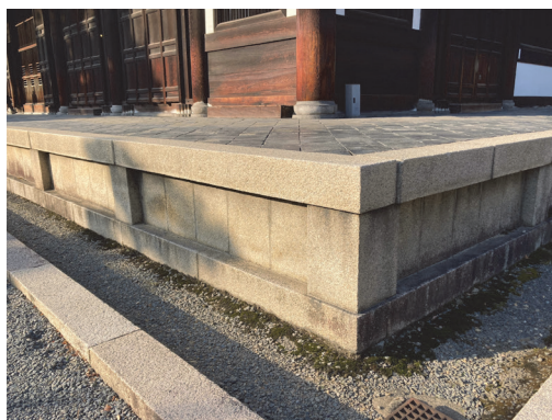
Fig. 2. Kiri-ishizumi masonry: precisely cut stone foundation used in Zen temples
