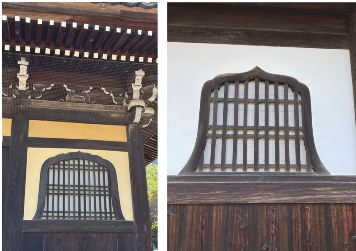
Fig. 9. Katōmado – distinctive wooden windows in Zen architecture, influenced by Indian design, featuring a bell-shaped curve and lattice grid with paper-covered shōji panels
