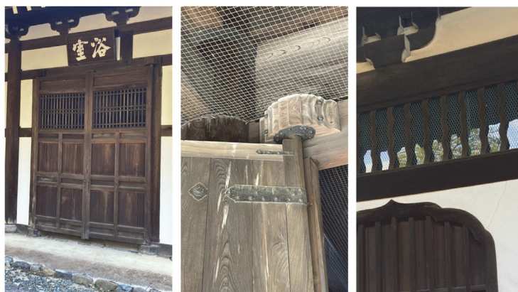
Fig. 10. Panel doors in Zen architecture, featuring lattice work, ornamental waraza projections, and wavy namigata renji slats above the door
