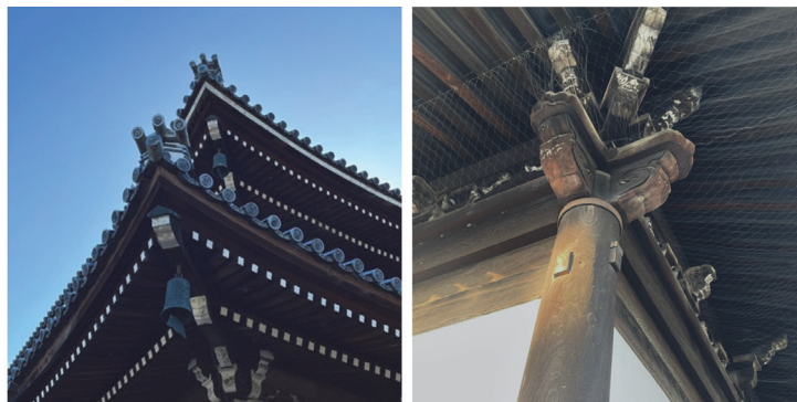
Fig. 11. Minimalist decoration in Zen architecture, featuring coloured paint on wooden construction elements (left) and kibana protrusions at the ends of beams (right)
