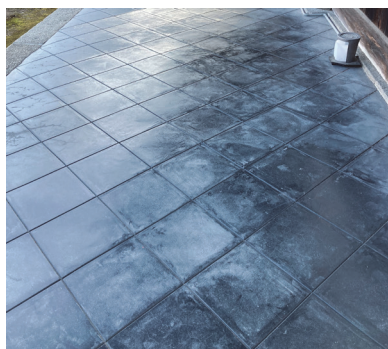
Fig. 3. Diagonal tiling ( shihanjiki ) in Zen temples, using square stone tiles laid at a 45° angle
