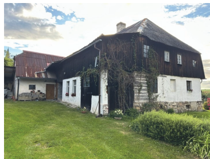
Fig. 4. Current state, south-east corner
