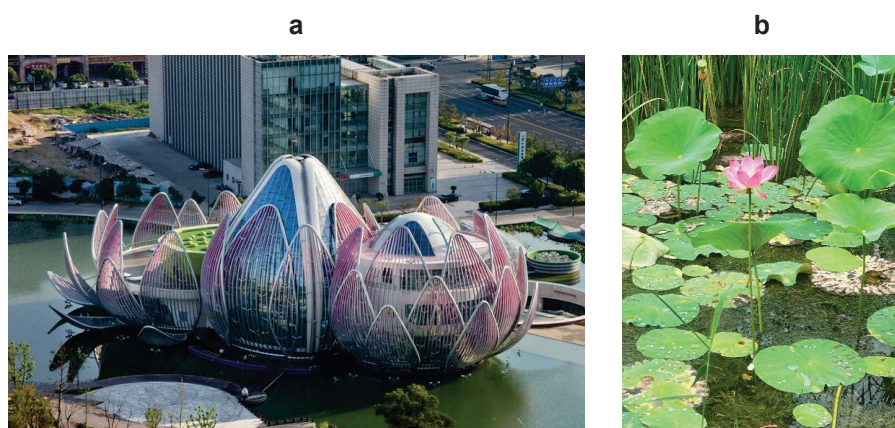
Fig. 2. Biomimetic architecture in China: a – Lotus Building in Changzhou, b – lotus flower as an architectural design inspiration
