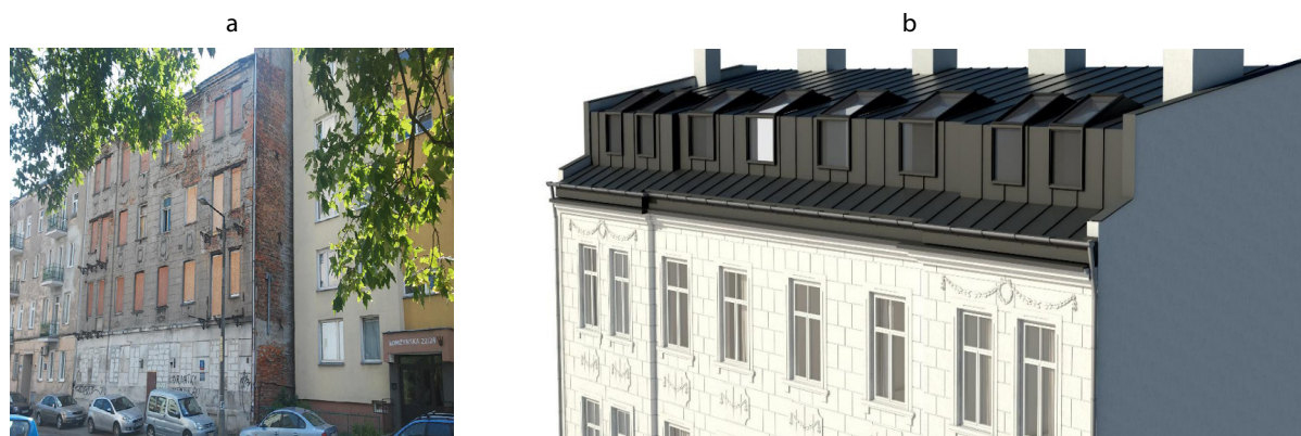
Fig. 7. Tenement house at Łomżyńska 26 in Warsaw – roof geometry before modernisation (a) and after modernisation (reconstruction project: architect Janusz Marchwiński). The shape of the roof, and the withdrawal of the window line, resulted from the street's visual analysis
