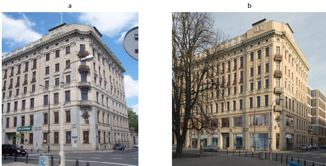
Fig. 1. Tenement house at Małachowskiego Square in Warsaw – the state before (a) and after renovation, which included shop windows installation on the 1 st floor (b)
