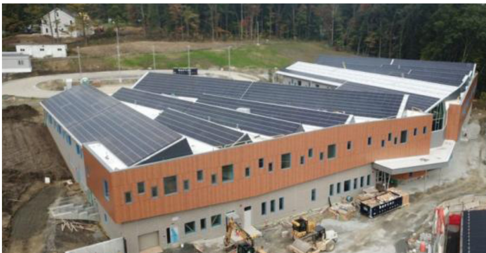
Fig. 2. Photovoltaic modules on the shed roof – Annie E. Fales Elementary School in Westborough, Massachusetts, USA Source: @HMFH Architects.
