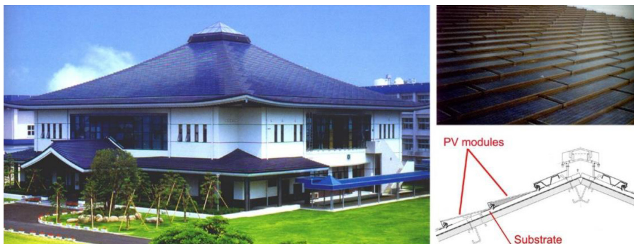
Fig. 1. Photovoltaic modules integrated with the gabled roof – Ho-Oh High School gymnasium building in Kagoshima, Japan
