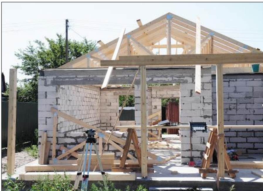
Fig. 7. Eco-friendly building constructed with autoclaved aerated concrete (AAC) blocks
