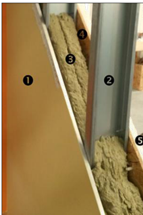
Fig. 5. Typical cross-sectional view of a wall in a lightweight frame construction: 1 – gypsum plasterboard; 2 – cold-formed steel profile; 3 – mineral wool; 4 – oriented strand board (OSB); 5 – external thermal insulation composite systems (ETICS) with thermoplastic expanded polystyrene (EPS)
