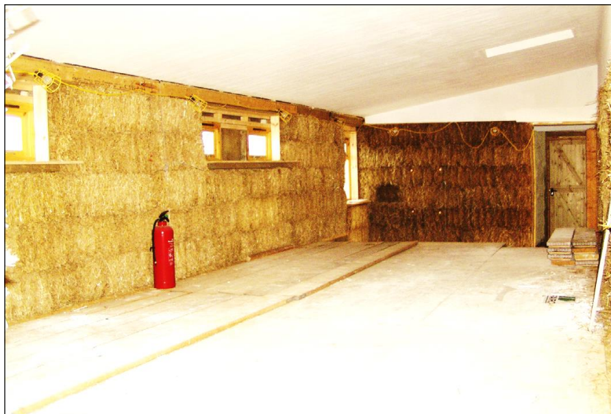
Fig. 9. Load-bearing wall constructed using straw bales
