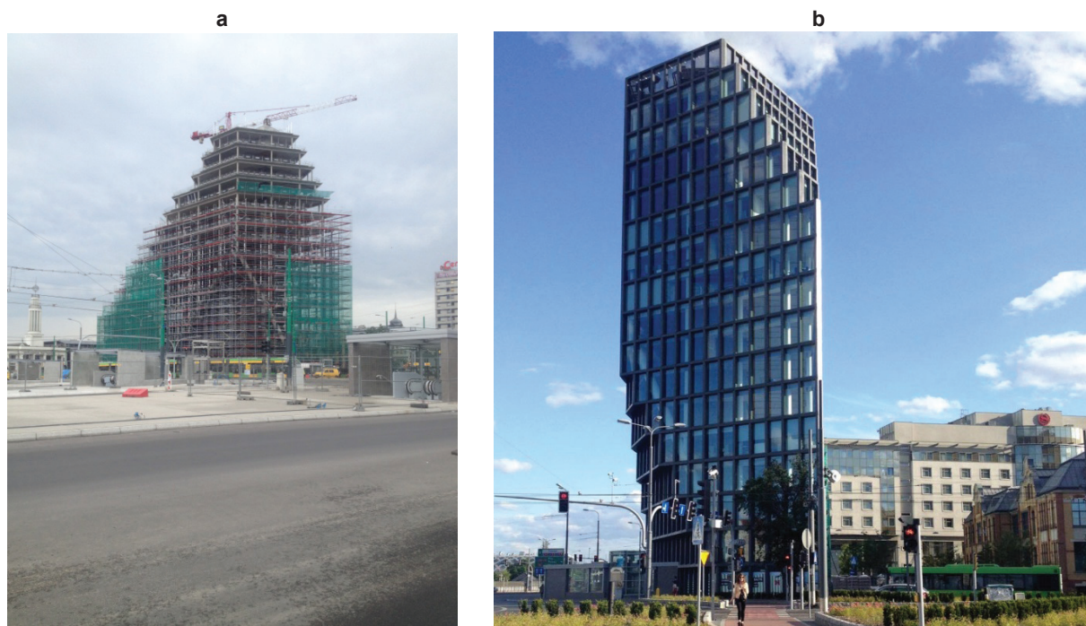
Fig. 2. The Bałtyk office building in Poznań (BREEAM certification level excellent): a – photo taken during the construction of the building, 2016; b – photo after the construction of the building was completed, 2017
