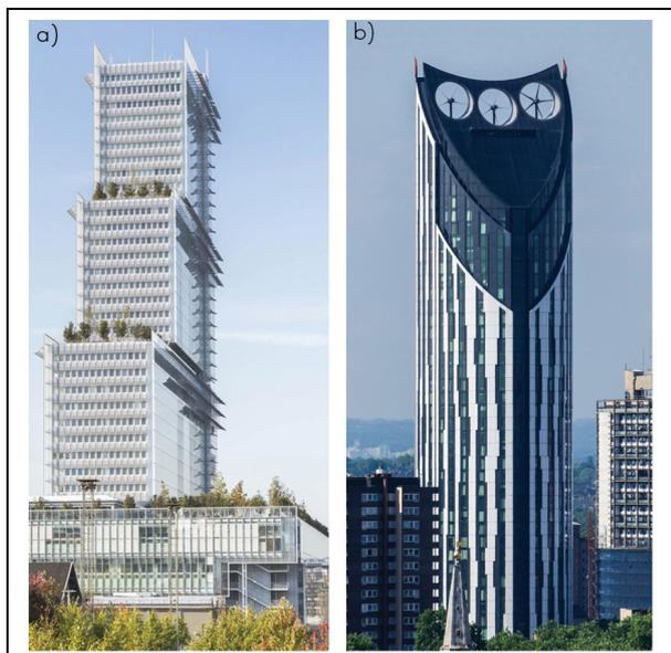
**Fig. 13.** Obtaining energy from natural resources: a – Tribunal de Paris, Paris, 2017 – inclined panels with PV cells; b – Strata building, London, 2010 – integrated wind turbines
