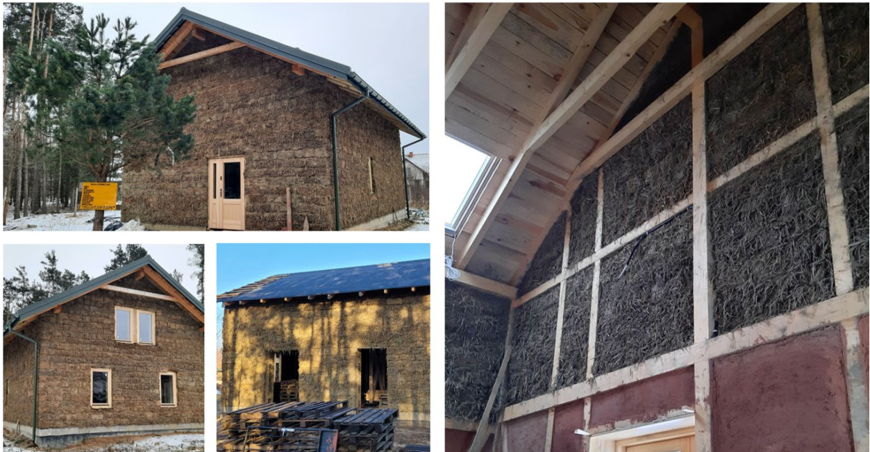
Fig. 5. A view of the half-timbered building in Jarzębia Łąka, Poland
