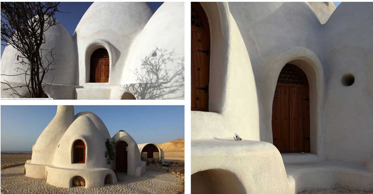
Fig. 7. House made of bags filled with earth and finished with clay plaster, Oman
