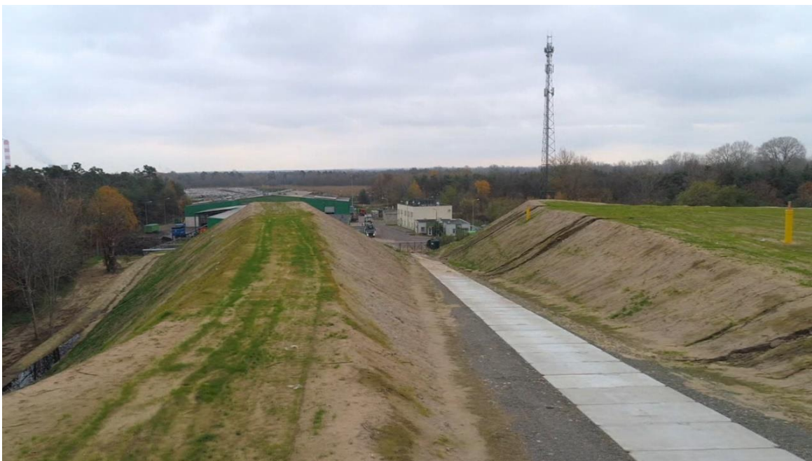
Fig. 8. View of the waste landfill in the Municipality of Puławy after recultivation – view from the south-eastern slope Source: own work.
