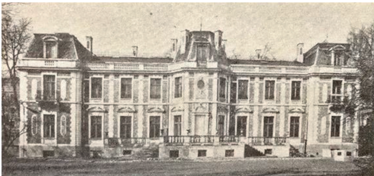
Fig. 8. Zamoyski Palace: garden façade with terrace on the axis
