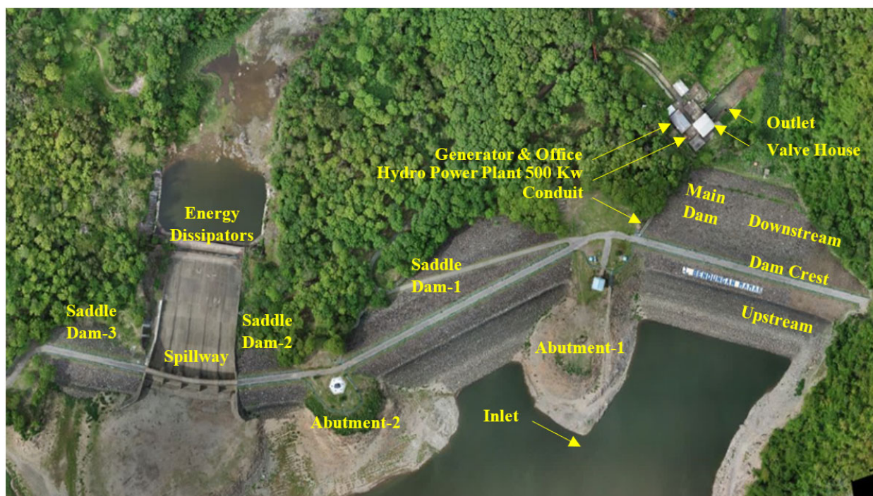
Fig. 1. Bird's view of the Mamak Dam
