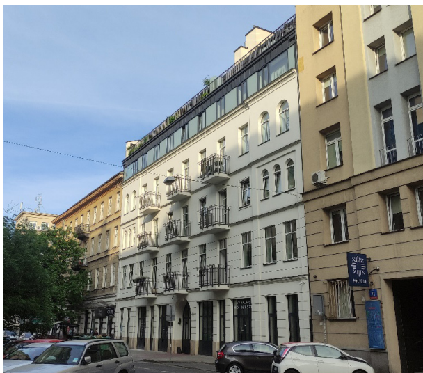
Fig. 9. The front elevation of the superstructured tenement house at Wilcza 19 in Warsaw in 2023. The façade in the strip of the top floor is stylistically different
