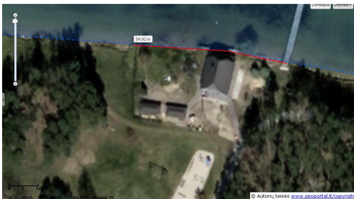
Fig. 1. The eroded coast of the lake Meteliai
