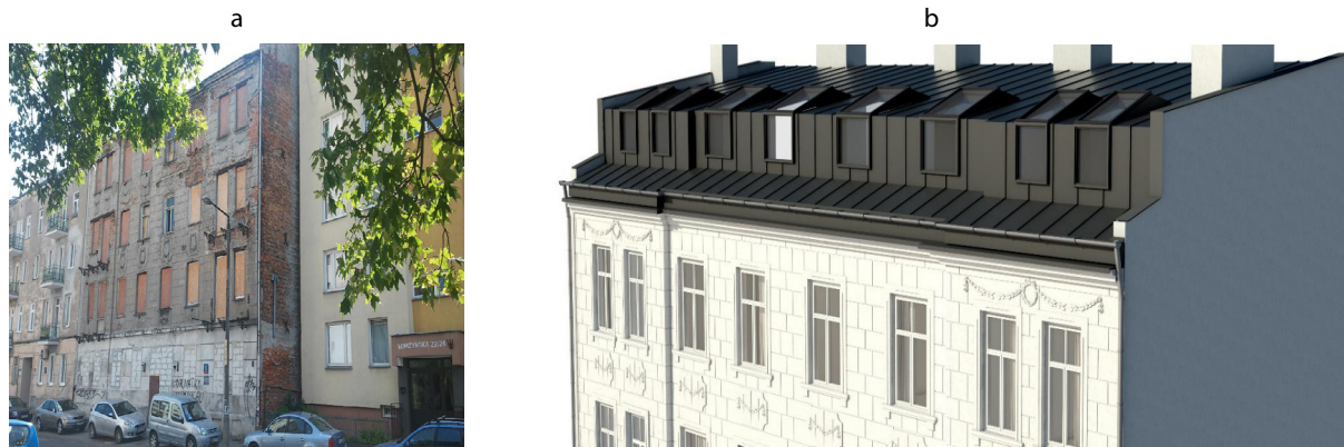
Fig. 7. Tenement house at Łomżyńska 26 in Warsaw – roof geometry before modernisation (a) and after modernisation (reconstruction project: architect Janusz Marchwiński). The shape of the roof, and the withdrawal of the window line, resulted from the street’s visual analysis
