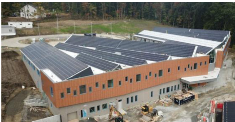
Fig. 2. Photovoltaic modules on the shed roof – Annie E. Fales Elementary School in Westborough, Massachusetts, USA Source: ©HMFH Architects.
