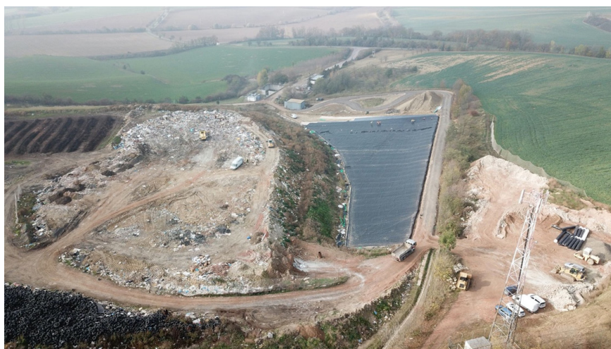
Fig. 2. Landfill body and landfill surrounding
