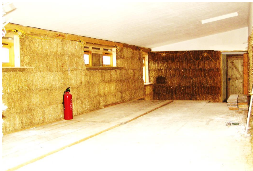
Fig. 9. Load-bearing wall constructed using straw bales
