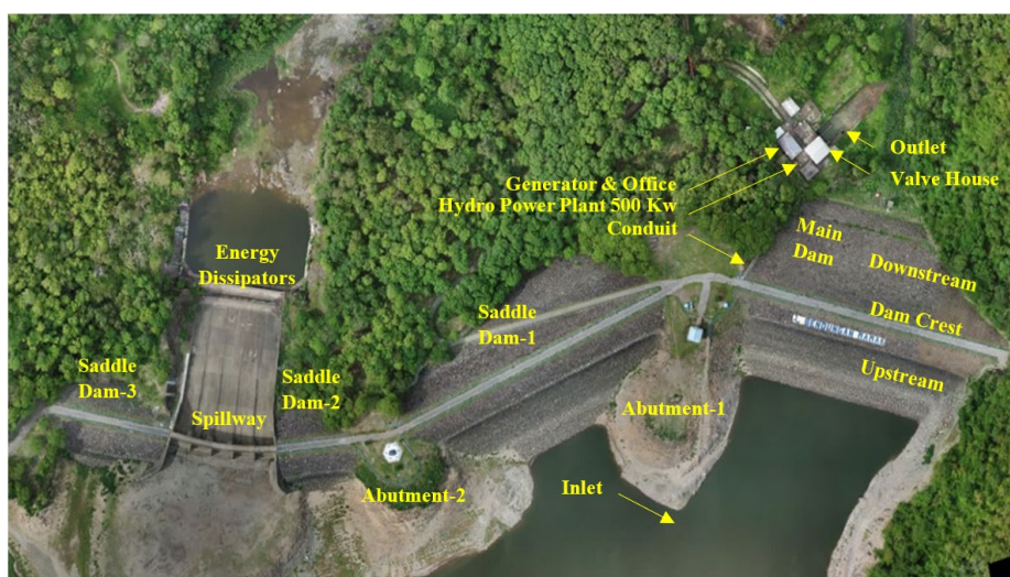
Fig. 2. Bird's view of the Mamak Dam
