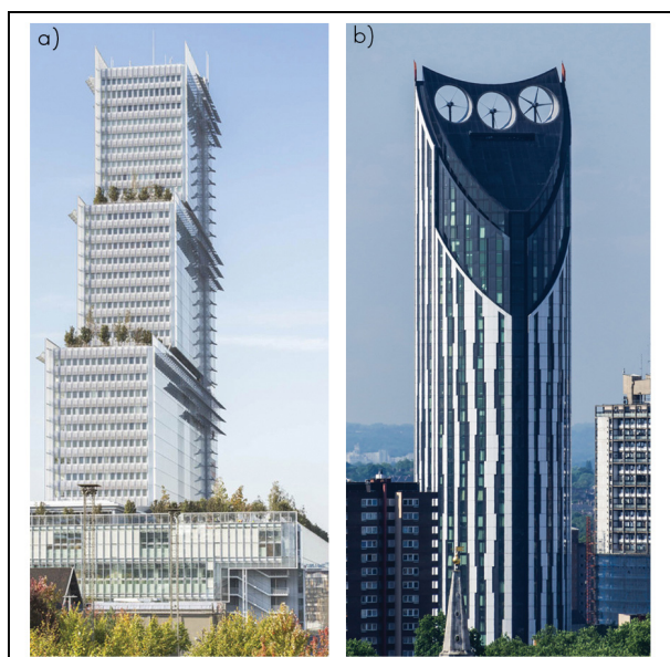
Fig. 13. Obtaining energy from natural resources: a – Tribunal de Paris, Paris, 2017 – inclined panels with PV cells; b – Strata building, London, 2010 – integrated wind turbines
