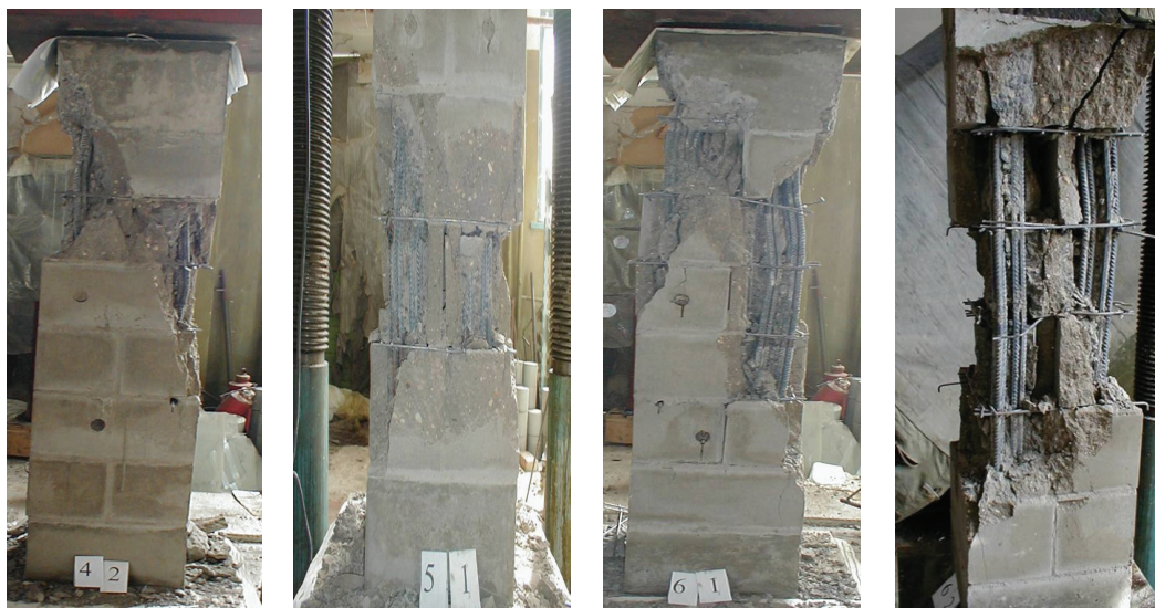
Fig. 6. The nature of the destruction of the columns
